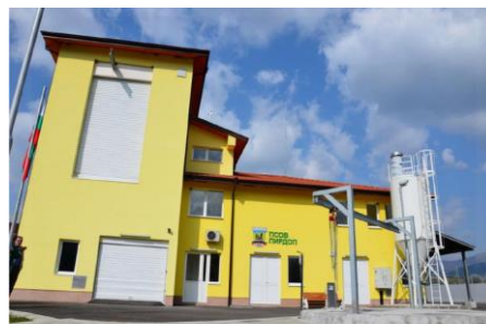
Pirdop wastewater treatment plant
